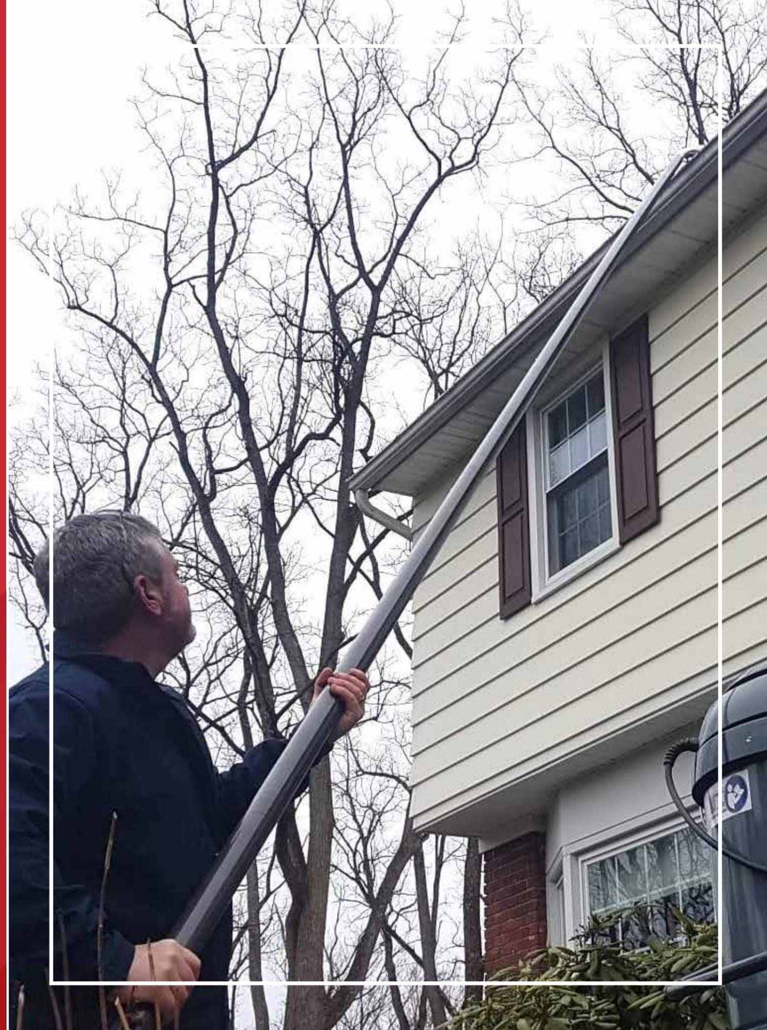
Working with carbon or aluminium reach poles near overhead electrically supply lines is extremely dangerous and has resulted in serious injury and loss of life.
